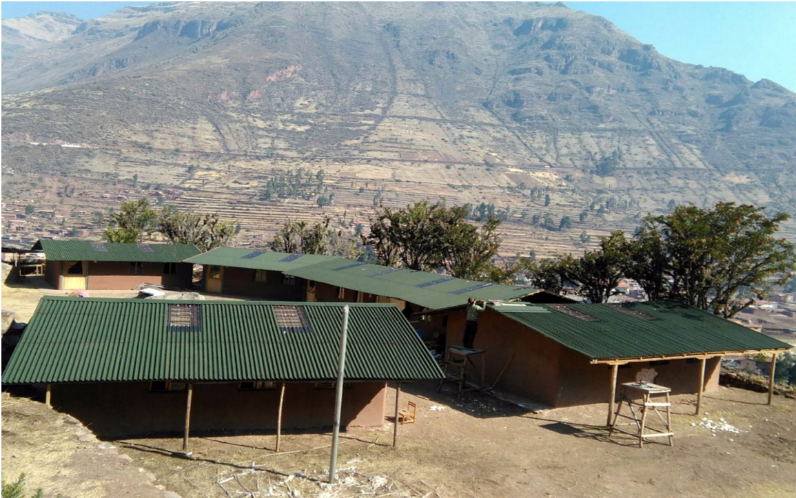
Our finished new roofs!
