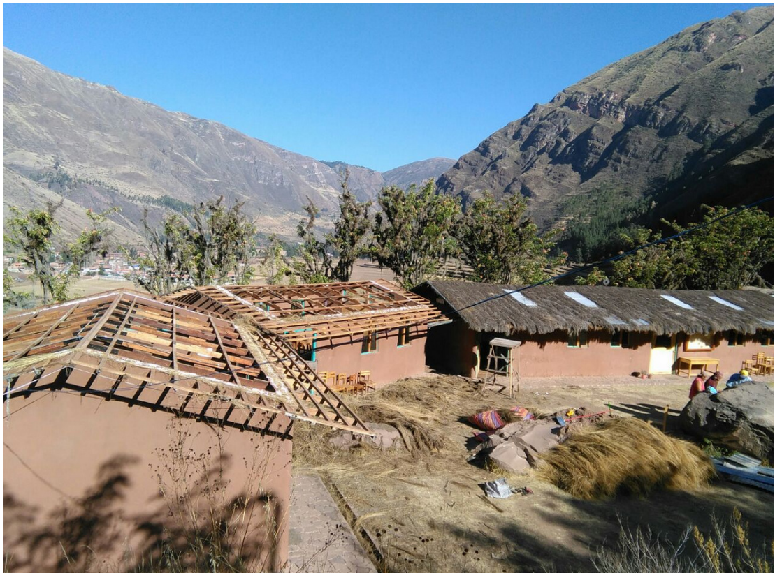
Removing the tin plates from the roofs.
