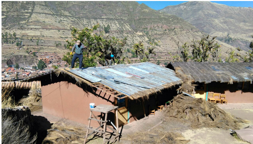
The first primary classroom – taking off the straw and nails (upper left hand corner).
